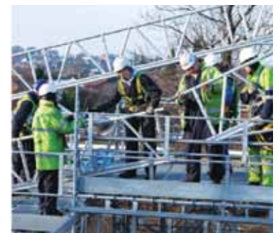
Training / Prebuild trial installation
